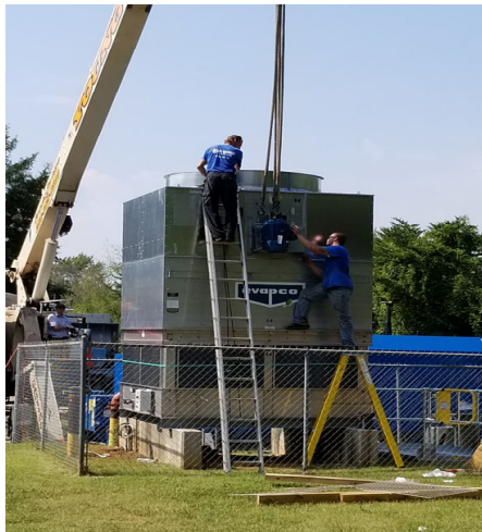
New cooling tower lowered into place at Tut Fann SVH.
